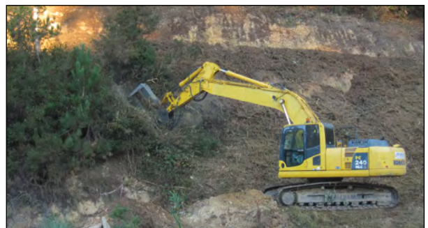
Easy access to difficult areas and slopes.
