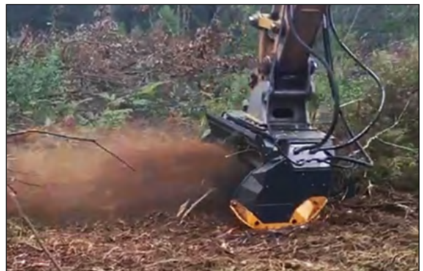
Land clearing for pipeline and hydro electric corridors.
